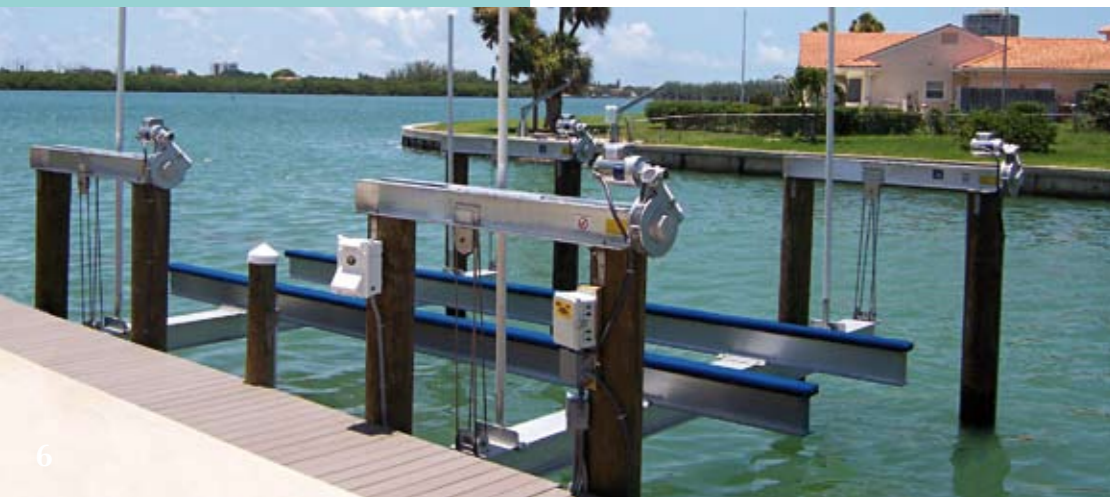
8 PILING BEAM LIFT
